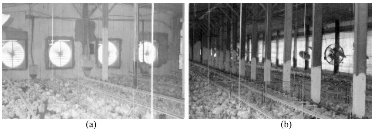
Figure 1. View of the exhausting fans (a) inside G2, and axial fans and side curtains (b) inside G1.
